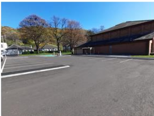
Carpark extension with tarmac finish, lining and lighting.
