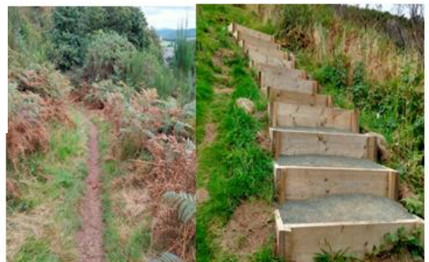
Improvement to existing section of path
