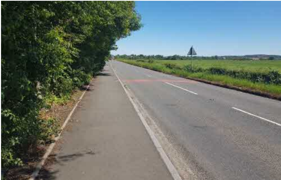
Photo 2.2 -View to East Along A91
