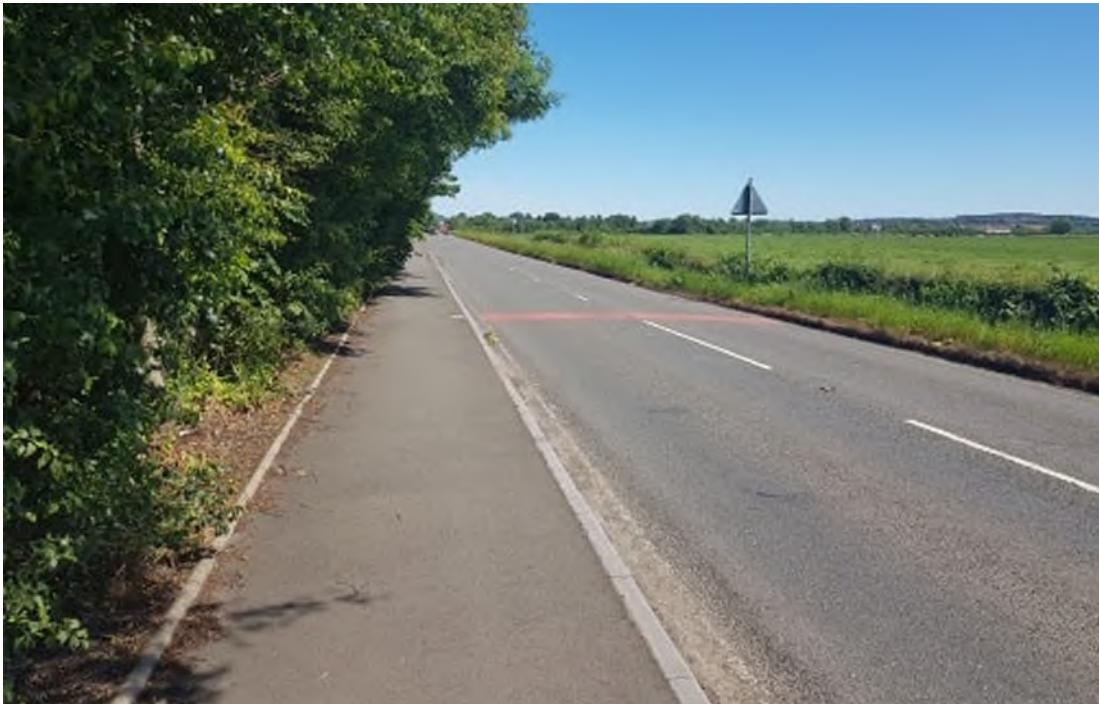
Photo 2.2 -View to East Along A91
