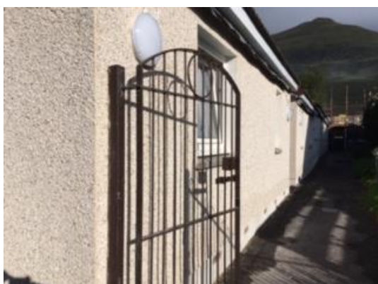
East entrance after roof and render
