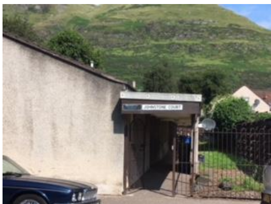
East entrance before works
