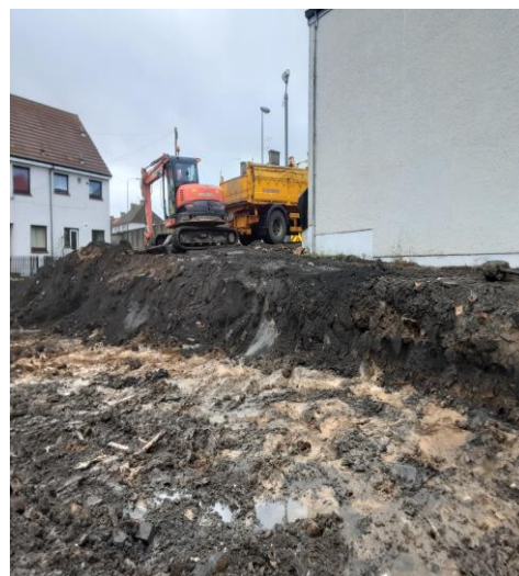
Excavation works ongoing
