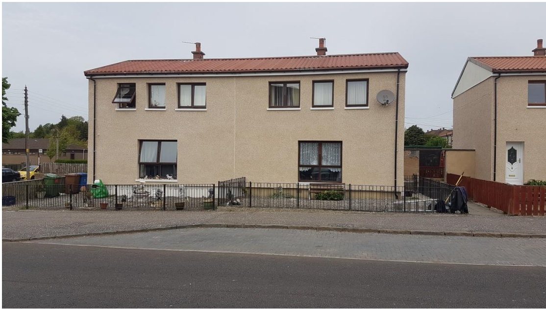
Non-Traditionally Built Upgrade – Clackmannan Lochies Road
