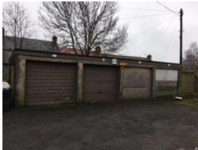
Lock ups prior to demolition
