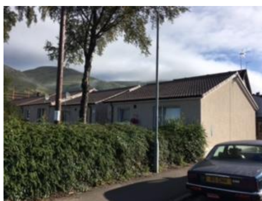
East view after roof and render works
