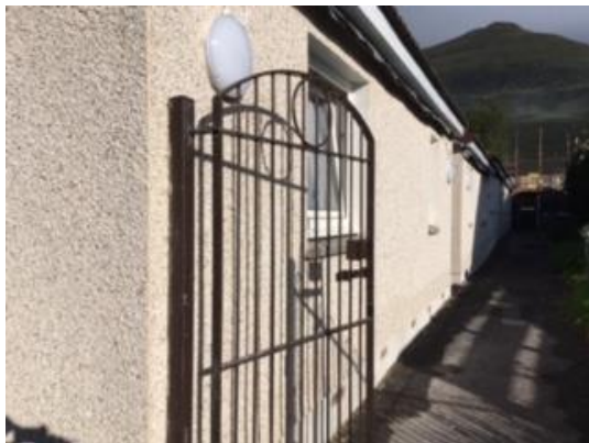
East entrance after roof and render
