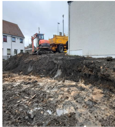
Excavation works ongoing
