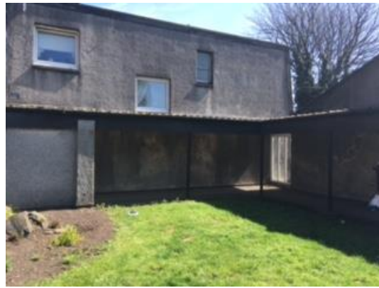
West of complex before works
