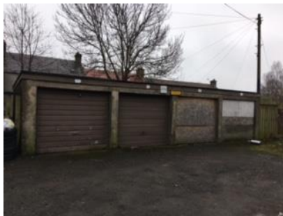
Lock ups prior to demolition
