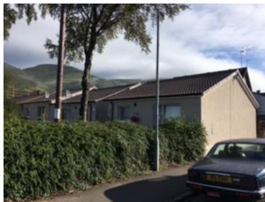
East view after roof and render works
