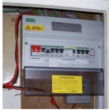
The new consumer unit will have switchable fuses (Miniature Circuit Breakers - MCB's) and a very sensitive fault detection switch (Residual Current Devise - RCD's or Residual Current Circuit Breaker – RCCB). The new consumer unit can help prevent injury or even death from electric shock.
