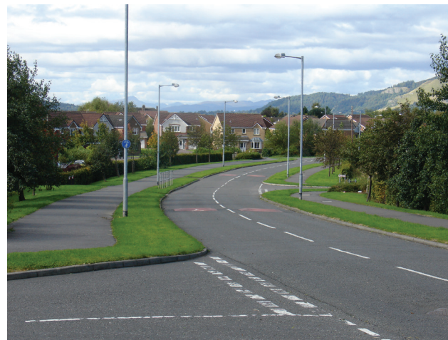
A wide road, with segregated footpath serving a residential development, but designed principally for car movement. The road width and geometry and segregation of pedestrians encourages higher vehicle speeds, necessitating speed cushions to be installed - Muirside Avenue, Tullibody
