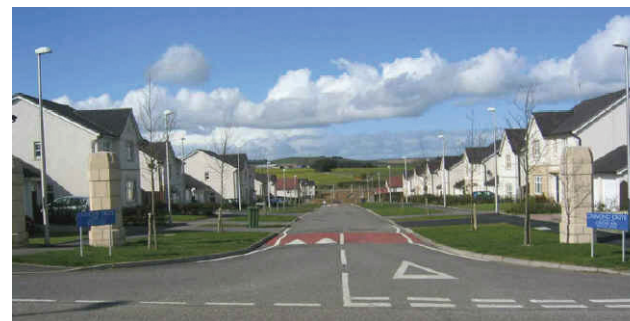
A street layout informed by overly rigid standards; large radius junction, over-dominant lighting columns, segregated footpath, standard driveways, and large building set-back which is an inefficient use of land
