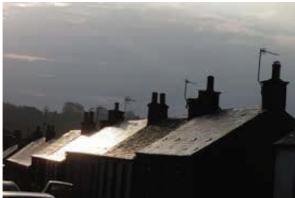
The stepping roofline enlivens street views in Stirling, Ochil, Hamilton and Hill Streets.
