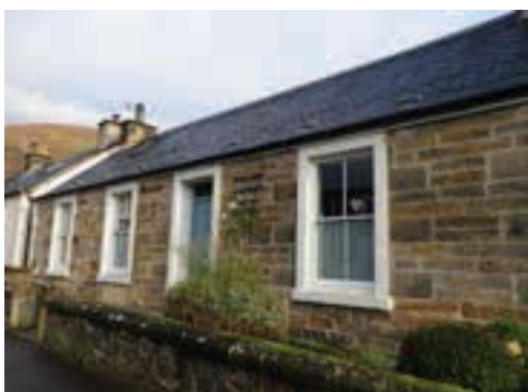
53 Ochil Street , c.1850. Single storey, 4-bay cottage. Timber two over two sash windows. Renewed slate roof with modern rooflight. Snecked tooled sandstone walls with painted window and door surrounds. Low boundary wall and small front garden to Ochil Street. Unlisted.
