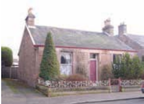
45 Hill Street , late 19 th Century. Single storey cottage in pinkish sandstone, tooled and coursed to front elevation, rubble to sides. Possibly original 2 over 2 timber sash windows. Scottish slate roof of diminishing courses with bracketed skewputs and moulded cornice at eaves. Chimney end stacks with decorative yellow clay pots. Low boundary wall topped with modern railings to street. Unlisted.
