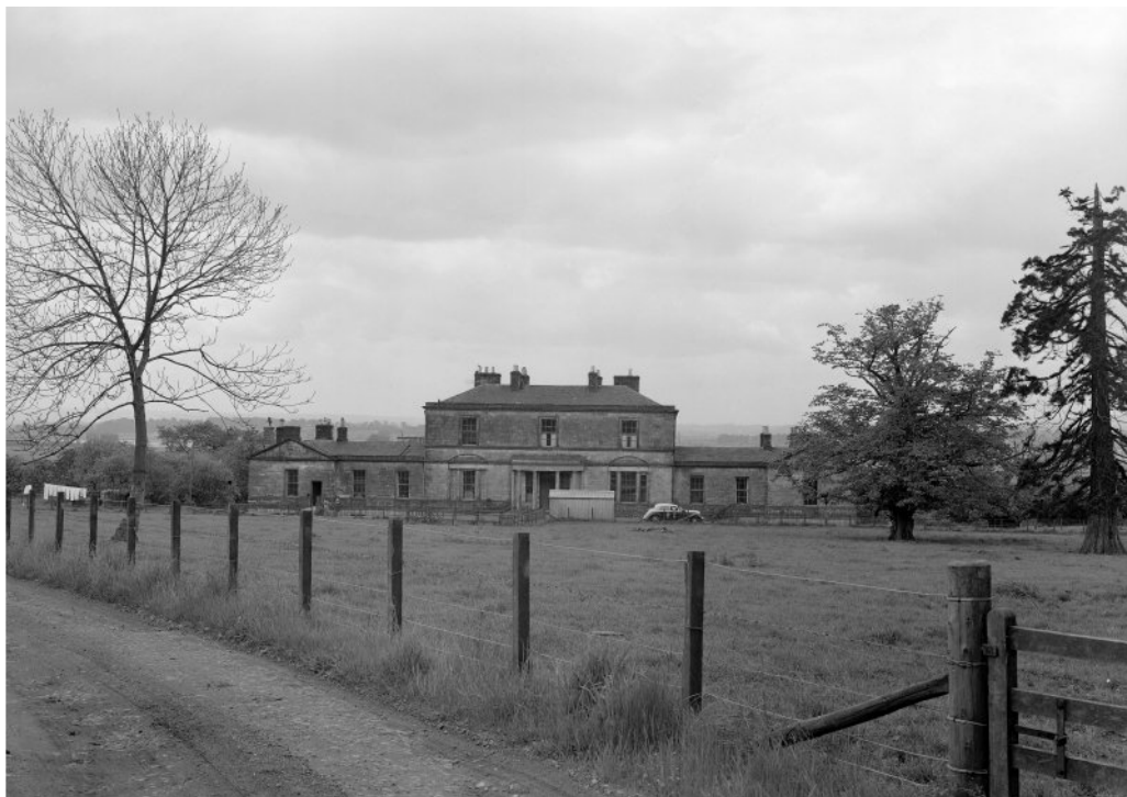
Kennet House Demolished in 1967
