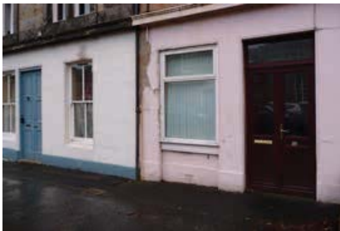
Insensitive uPVC replacement windows and doors on McNabb Street.
