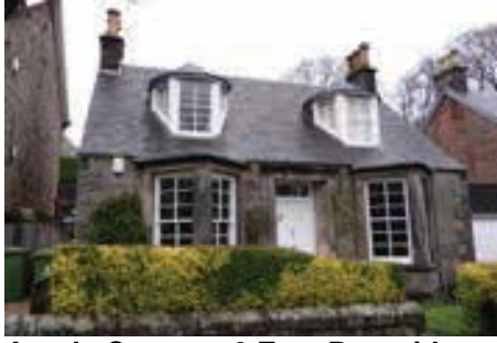
Argyle Cottage, 6 East Burnside , c.1835 One and a half storey cottage of grey ashlar stone with pitched slate roof. Triangular bay windows either side of a central door and canted dormers containing lying panes. Low front boundary wall with hedge forms boundary to the road. Category B-listed.
