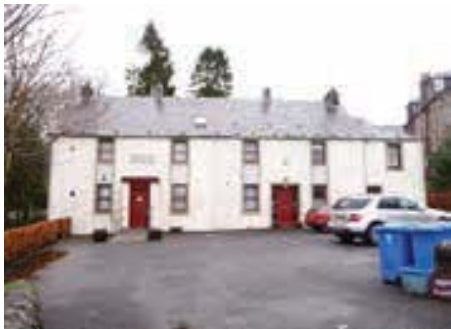
Dollar Museum, built 1820 as a woollen mill. Walls covered in painted harl with pitched slate roof. Converted to a hall in the late 19 th Century when the top floor was removed and the windows of the ground and first floors were joined to create vertical openings. These openings were partly built up in 1991 when the building was adapted to a museum. Category C-listed.
