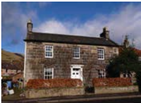
86 Bridge Street, c.1820. Symmetrical well proportioned house with a central door and pilastered surround with rosettes. Built as Bridge Street began to be feued by the Harviestoun Estate in the 1820s. Several similar buildings survive along Bridge Street from the same period, such as the Railway Tavern, which features the same door surround. Front boundary wall with hedge forms the boundary to the road. Category B-listed.
