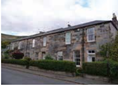
Charlotte Place, 4-8 Harviestoun Road, c.1820. A symmetrical two-storey ashlar row with a hipped slate roof and a central name stone. A low boundary wall to the front is topped with a hedge. Named after one of the daughters of Leishman of Broomrigg who must have put money into the building. Another Leishman daughter is commemorated in Helen Place, further west along Harviestoun Road. Category C-listed.
