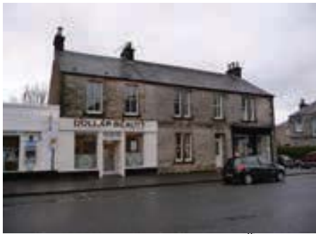
47-53 Bridge Street , late 19 th Century two-storey commercial property in grey ashlar, with a pitched slate roof. Retail at each end of ground floor with residential above. Some paired narrow sash windows. To the right a good surviving 19 th Century shopfront, painted black with scrolled console brackets and a splayed entrance lobby with narrow cast-iron columns. Category C-listed.
