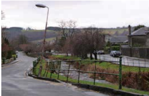
The Burnside Regeneration Project aims to enhance the overall environment of the Dollar Burn.
