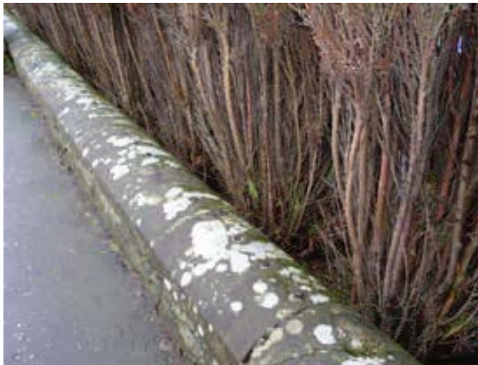
Low boundary wall in Bridge Street
