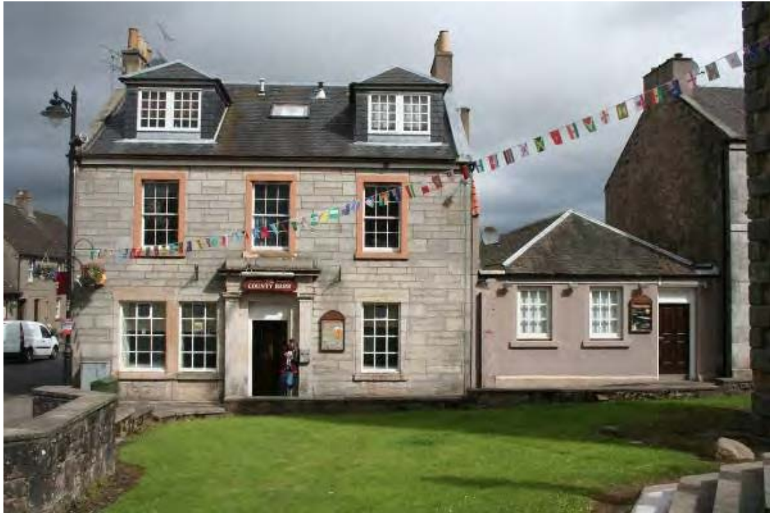
Figure 2-1: Clackmannan, Country Barr, Main Street, August 2014 (Peter Drummond Architects)
