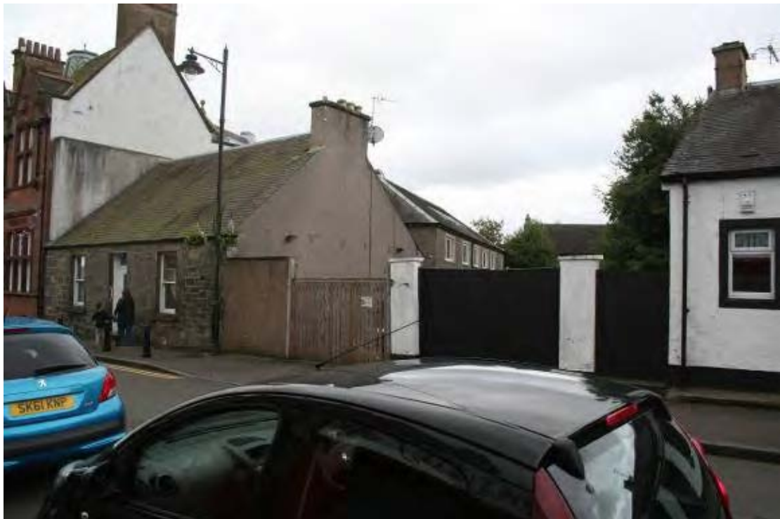
Figure 4-29: Clackmannan, Gap site at 56-62 Main Street, August 2014 (Peter Drummond Architects)
