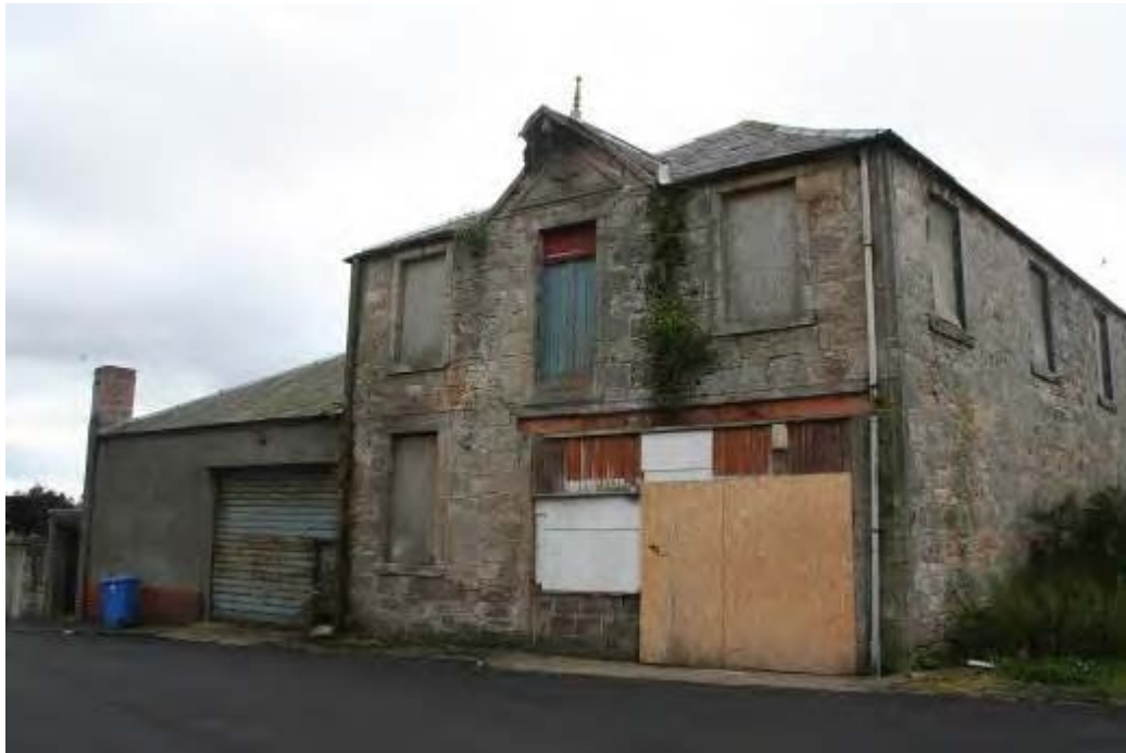
Figure 4-10: Clackmannan Co-operative Building, North Street – August 2014 (Peter Drummond Architects)
