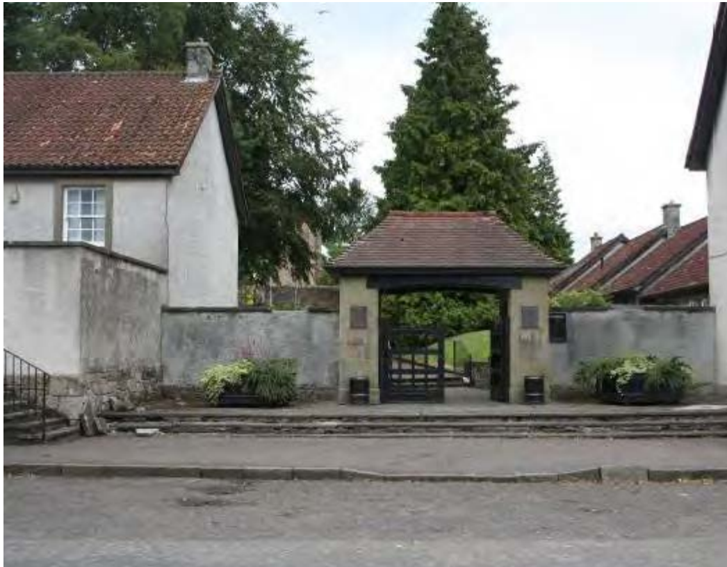
Figure 5-2: Clackmannan, lych gate, Port Street, August 2014 (Peter Drummond Architects)
