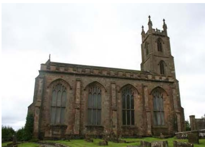
Figure 4-15: Clackmannan, Clackmannan Parish Church, High Street, August 2014 (Peter Drummond Architects)
