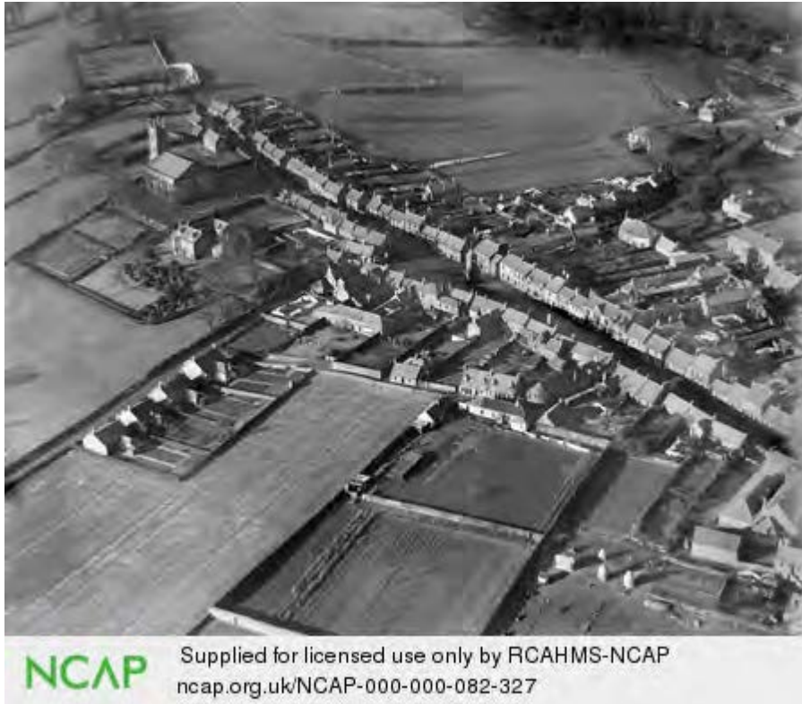
Figure 2-4: Aerial view of Clackmannan in 1928 (© RCAHMS)
