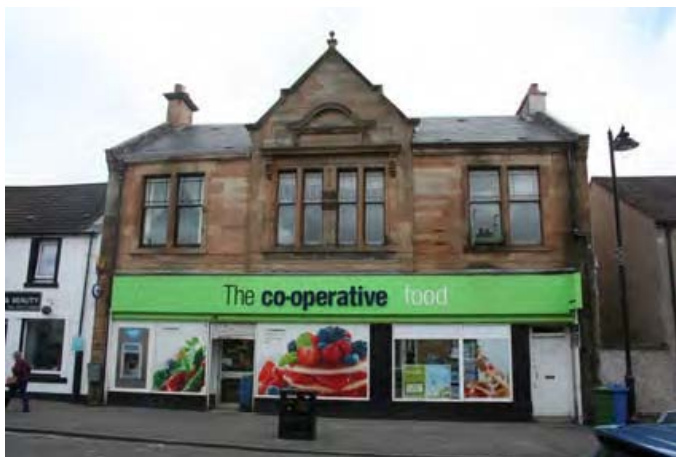
Figure 4-25: The Co-operative Food, 23-25 Main Street, August 2014 (Peter Drummond Architects)
