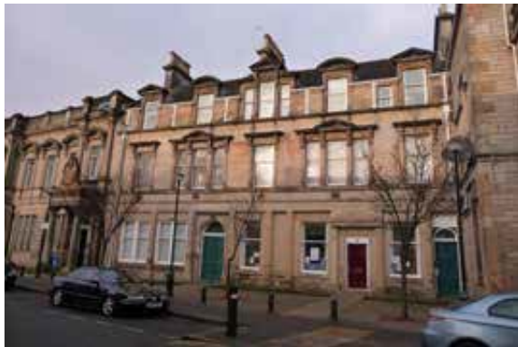
The public realm outside the former Burgh Chambers has potential for improvement
