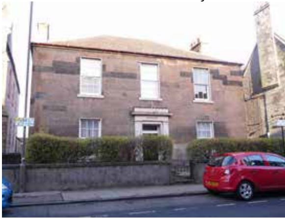
Below: Moncrieff House is currently on the Buildings at Risk Register for Scotland.
