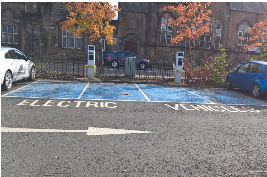
Figure 2.2 - Public electric vehicle charging bay in Greenside Street car park, Alloa
