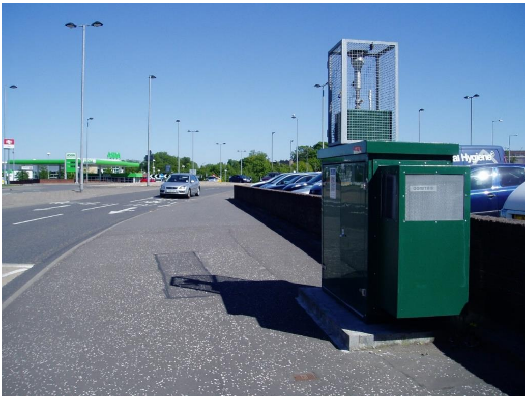
Figure 3.1 – Automatic Monitoring Site - King Street, Alloa
