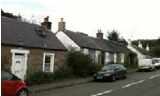
Main Street features low one-storey cottages set directly on the roadside
