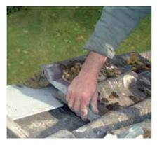
If necessary new roof valleys are formed to seal the roof where roof faces join. The roof valleys help to carry rainwater away from the roof.
